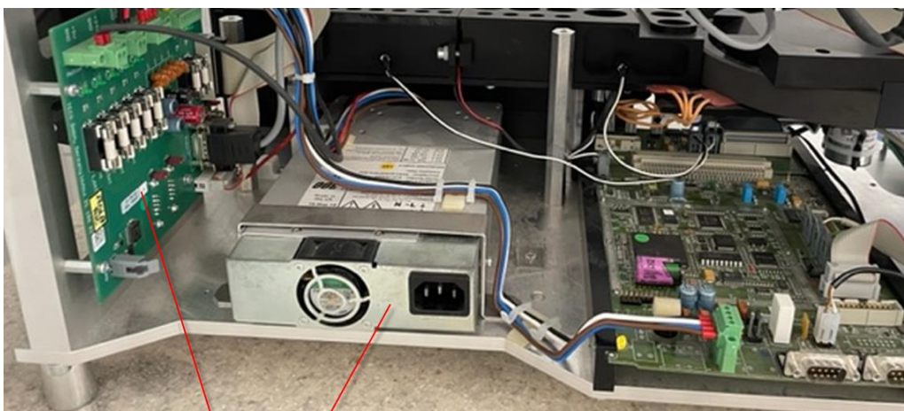
mount new power board and power supply
